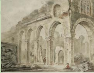
2 Demolition of Norwich Cathedral Infirmery John Crome, c1804. NWHCM : 1922.135.886
